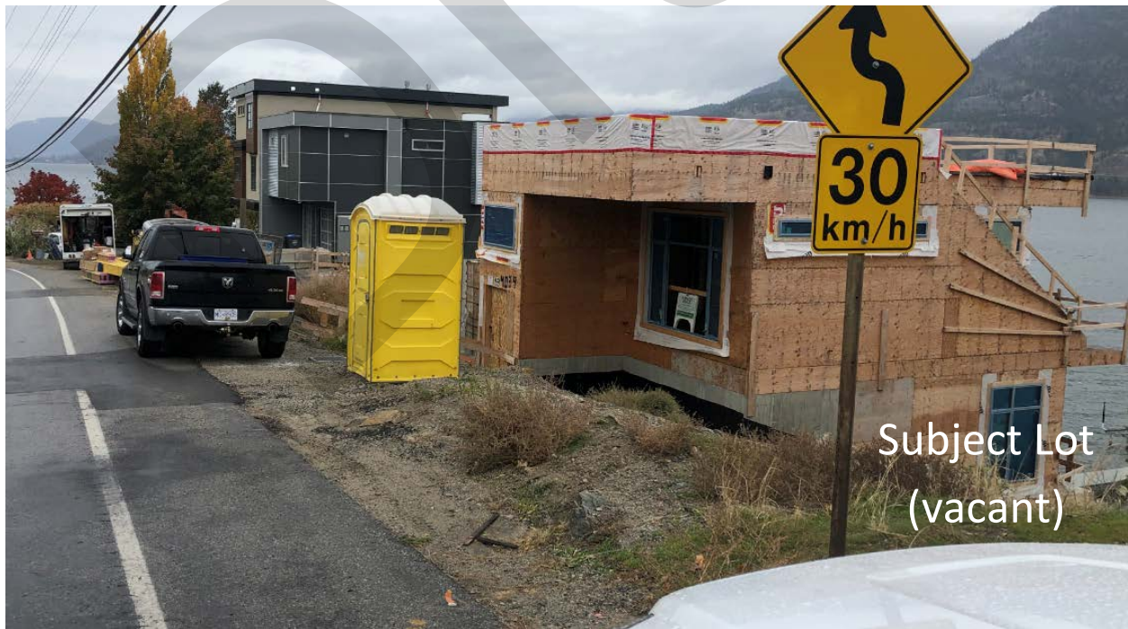
Figure 2: Image of other lots under various levels of completion along Lakeside Road
